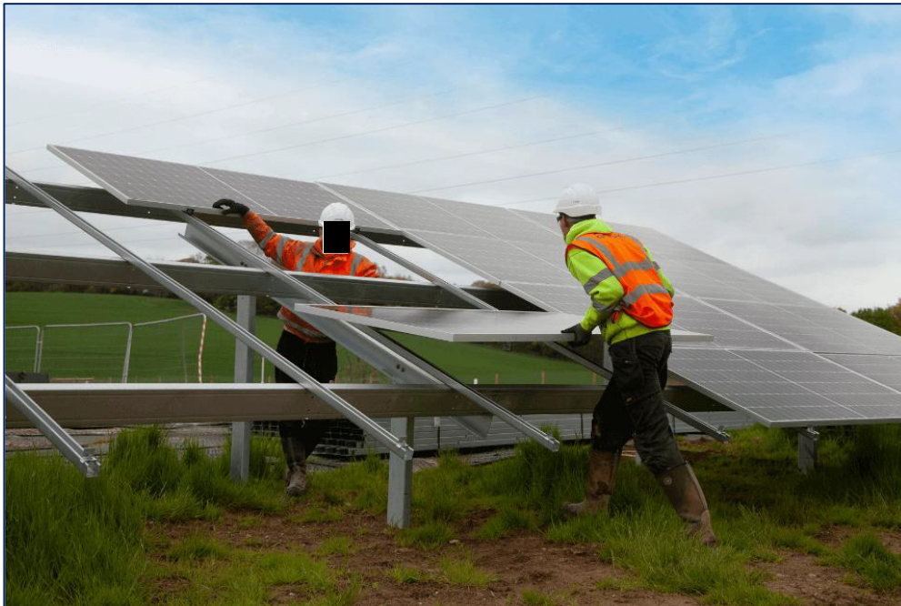
Plate 12-24 PV module installation (Ref. 12-16)
