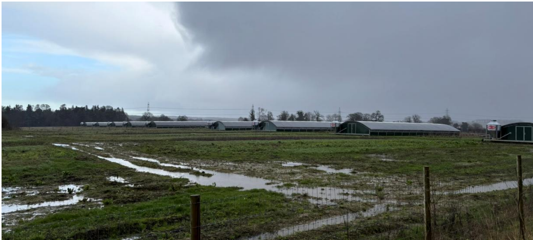
Plate 12-16 Areas of surface water ponding and generation
