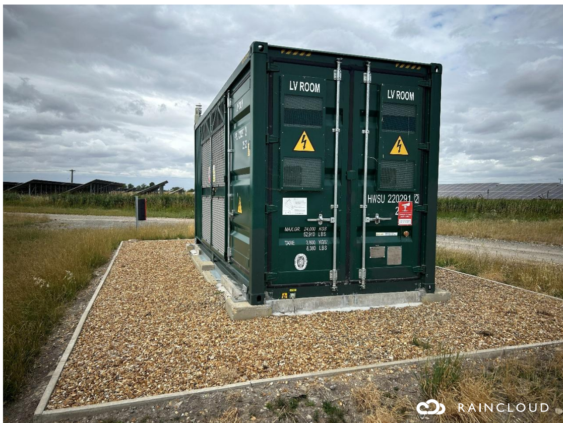
Plate 12-33 Conversion unit gravel surround
